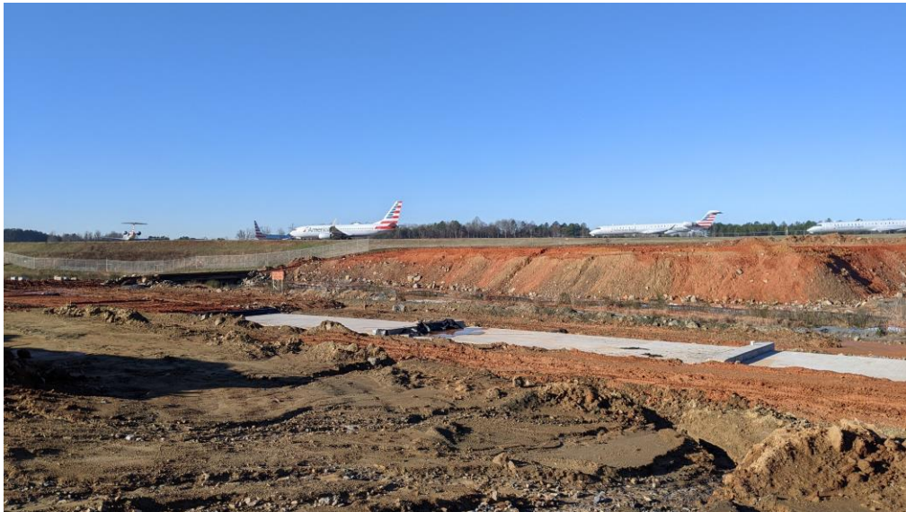
Site for Deicing pad & Taxi Lane – Charlotte Douglas International Airport, NC
